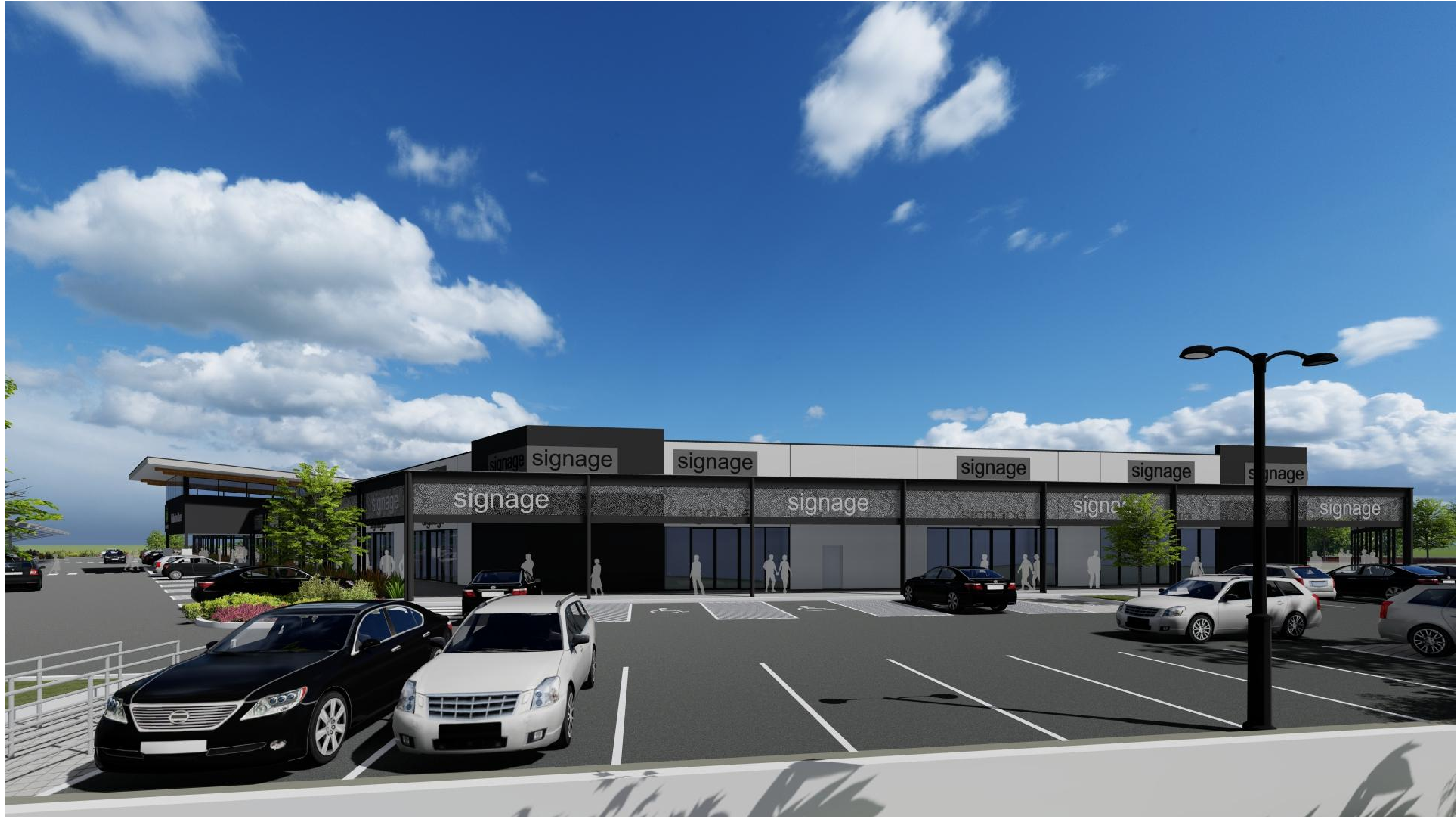
SOUTH-EASTERN / VERANDAH VIEW
